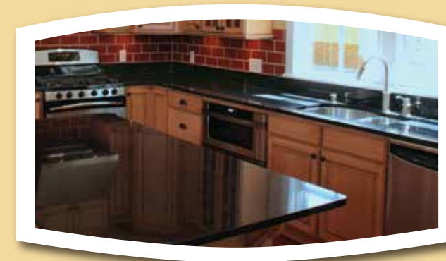
Granite counter with stainless steel sink single bowl with single drain board of reputed make.
