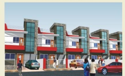
Tejaji Nagar, By-pass, Khandwa Road, Indore
